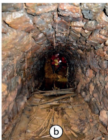
Figure 6: Types of tunnel cross-sections: a. section in tunnel 2, with enlargement in stratified lava flows; b. tunnel 6 entrance, lined with andesite blocks; c. weathered bedrock with extended limonite deposits in tunnel 6.
