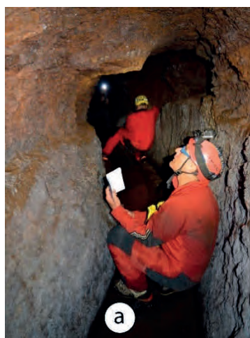
Figure 6: Types of tunnel cross-sections: a. section in tunnel 2, with enlargement in stratified lava flows; b. tunnel 6 entrance, lined with andesite blocks; c. weathered bedrock with extended limonite deposits in tunnel 6.
