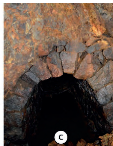
Figure 6: Types of tunnel cross-sections: a. section in tunnel 2, with enlargement in stratified lava flows; b. tunnel 6 entrance, lined with andesite blocks; c. weathered bedrock with extended limonite deposits in tunnel 6.
